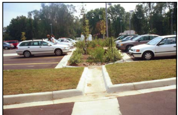
After: Bioswale Installed in Parking Lot at Mallett's Creek Library
