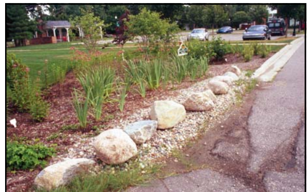
Lathrup Village Community Rain Garden – Rock Infiltration Sump Installed to Remove Water Quickly
